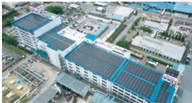
Mimaki Engineering's Kazawa Factory, which has introduced a solar power generation system (on-site PPA).
